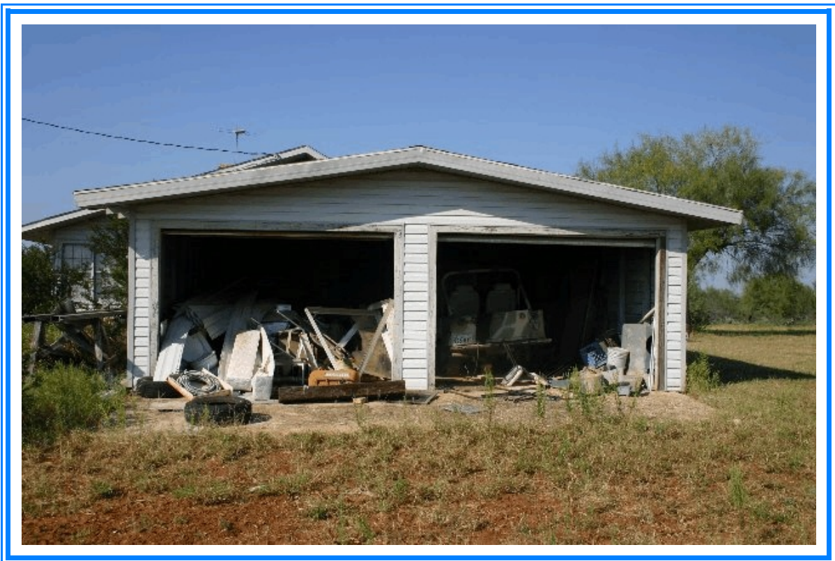
FRONT VIEW OF GARAGE AT THE GRANDMOTHER'S HOUSE
