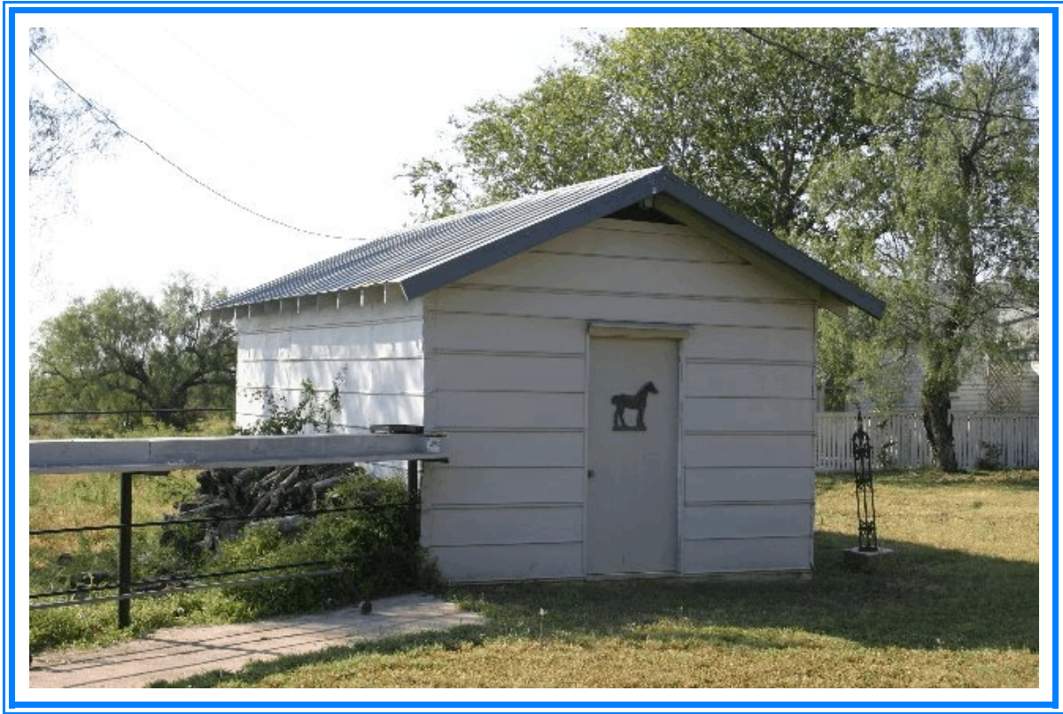
FRONT AND SIDE VIEW OF THE TACK ROOM
