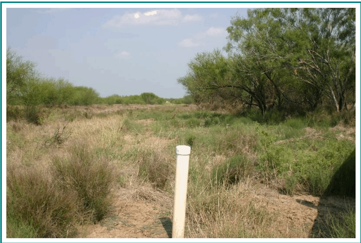
VIEW OF UNDERGROUND WATER LINE
