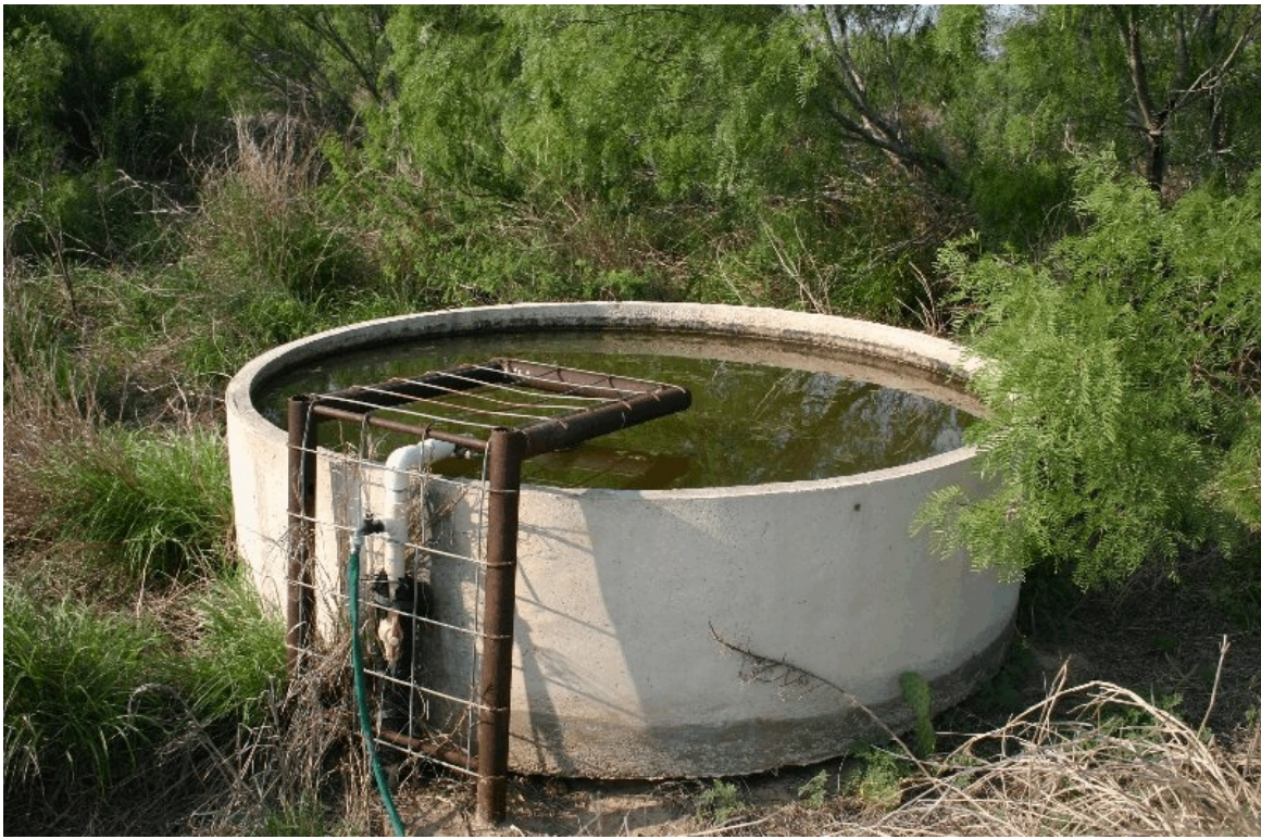
VIEW OF CONCRETE WATER TROUGH
